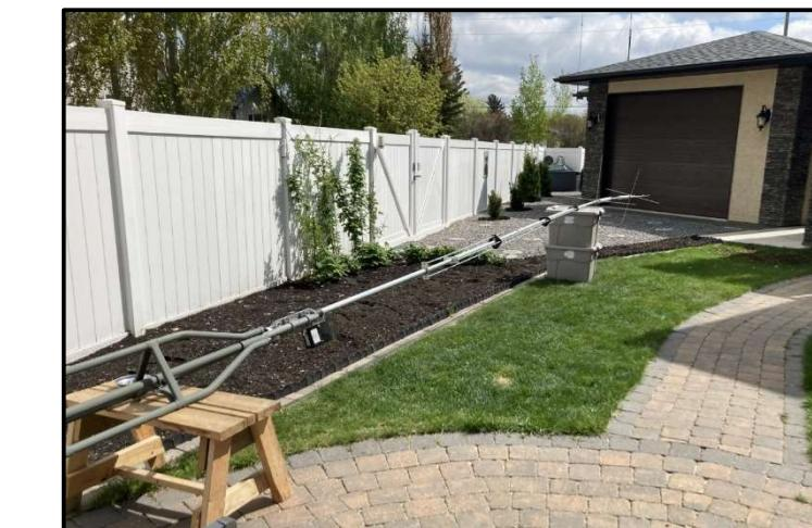
The antenna assembly can be easily raised and lowered using a hand winch assembly (not shown). This tilting tower design eliminates the need for any ladder or scaffolding during antenna maintenance.
